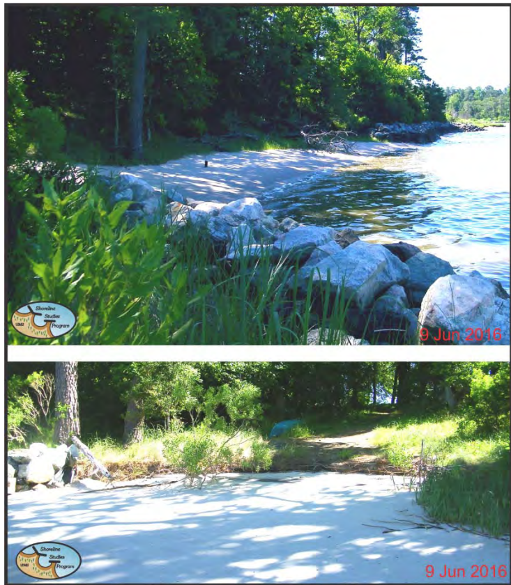
Figure 10. The sandy beach between the high continuous sill and rock revetment has a sloped bank making the area accessible.
