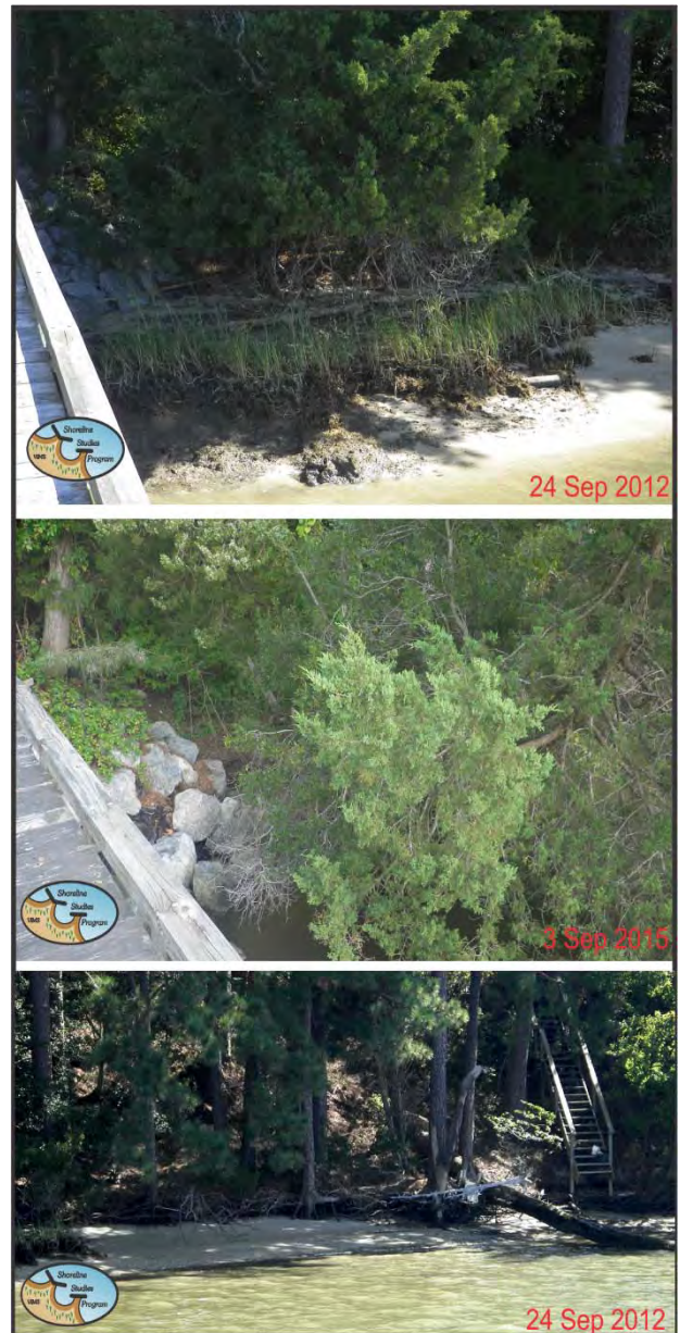
Figure 8. Marsh loss at the site. Top: In 2012, several areas of marsh still existed in front of the bank, however, it was eroding quickly. Middle: By 2015, the marsh in front of the bank was completely gone and several of the trees on the shoreline had fallen due to erosion. Bottom: Concern for archaeology in the actively eroding bank led to the placement of a gapped sill living shoreline system.
