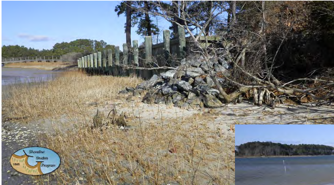
South End: Revetment placed along the eroding upland with a narrow marsh in front.
