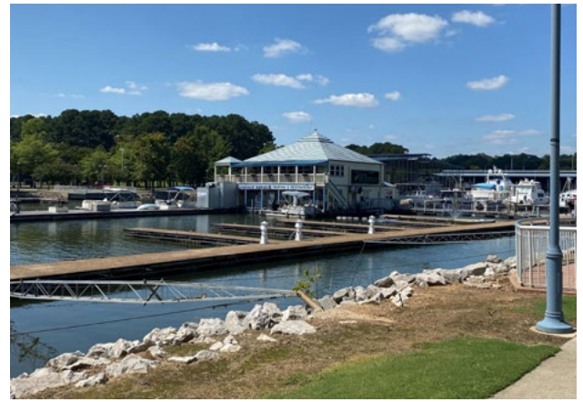
Florence Harbor Marina, Alabama, used BIG funds to renovate an existing 460-foot transient dock by adding new dockside power pedestals, providing water service, and replacing worn decking and flotation. (credit: Alabama Department of Environmental Management)
