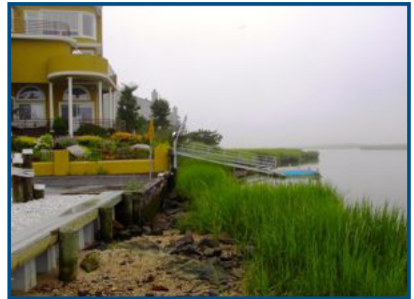
This tidal marsh has been prevented from migrating landward by a sea wall, an example of "shoreline squeeze."
