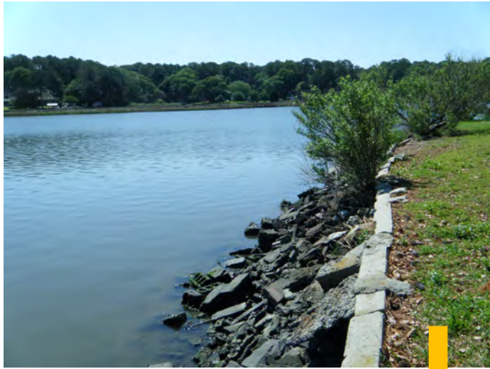
Failing bulkhead
