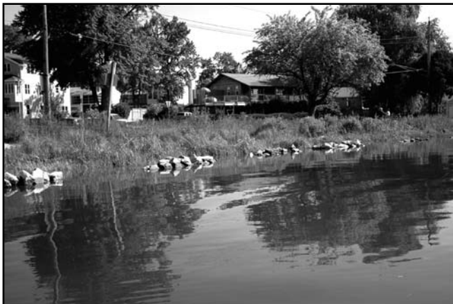
Figure 2. 12-foot long sills with 6-foot windows at the living shoreline site in Glebe Bay, South River, Maryland.
