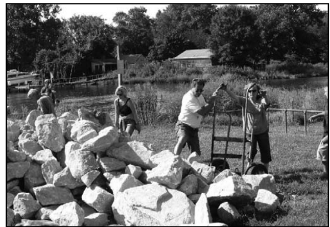
Figure 3. Contribution of volunteer labor: 200 volunteers contributed 800 hours to construction of the living shoreline in Glebe Bay, South River, Maryland.
