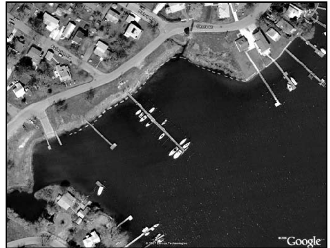
Figure 1. Placement of 33 segmented stone sills to create a living shoreline along 750 linear feet of shoreline in Glebe Bay, South River, Maryland
